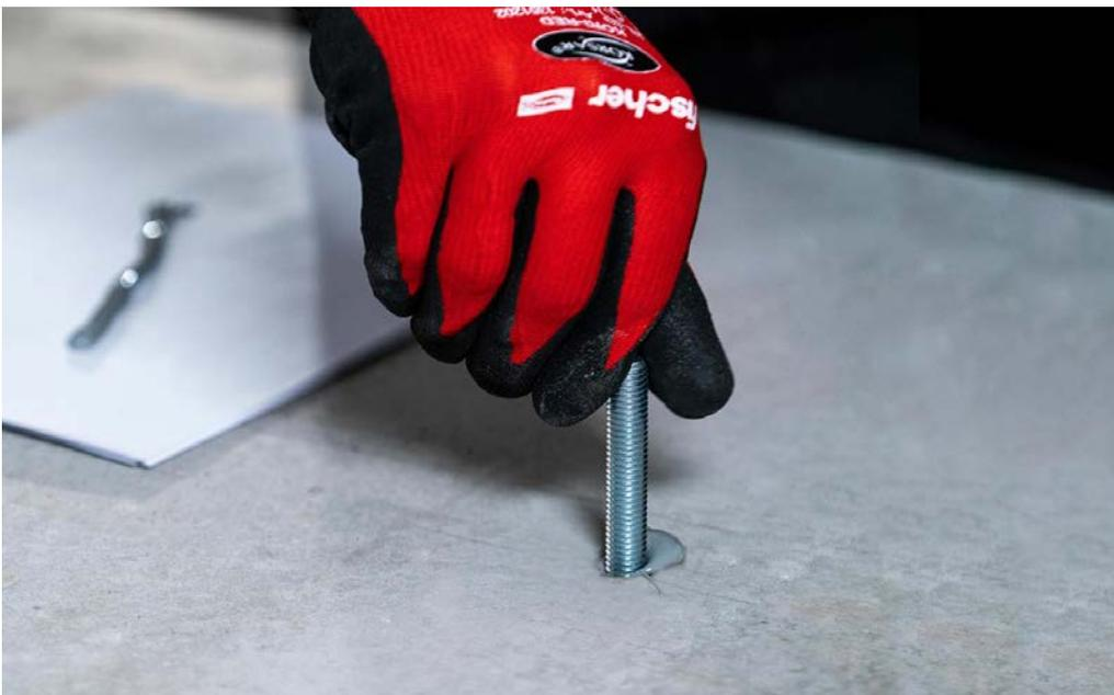
When using injection systems, anchor rods are mounted into the mortar-filled drill hole by hand with a slight rotary movement.
